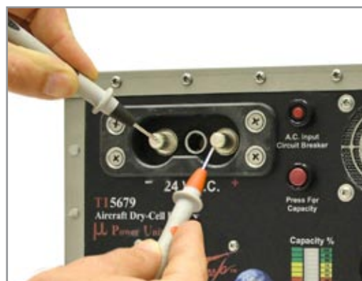
Figure 3.9.3 – Testing DC Receptacle
