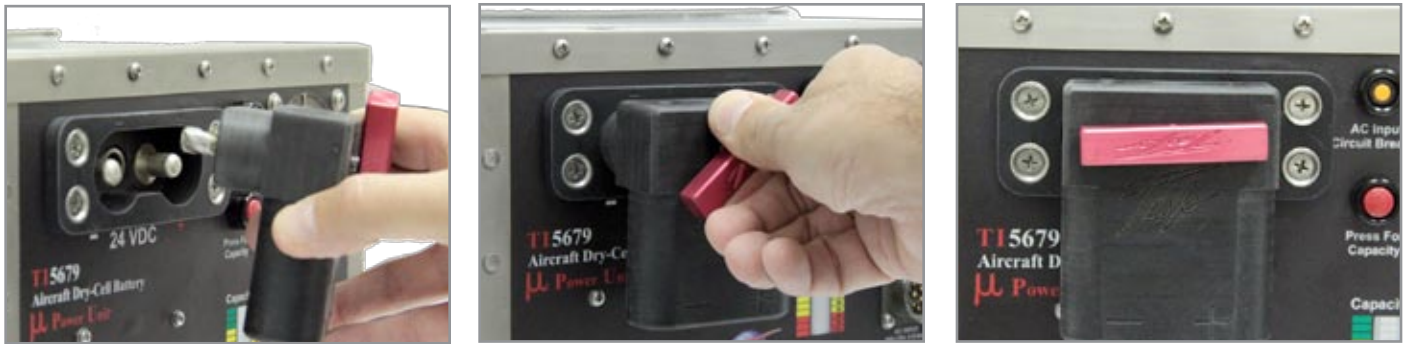
Figure 3.10.1 Attaching dc power cable to TI5679 MPU-24
