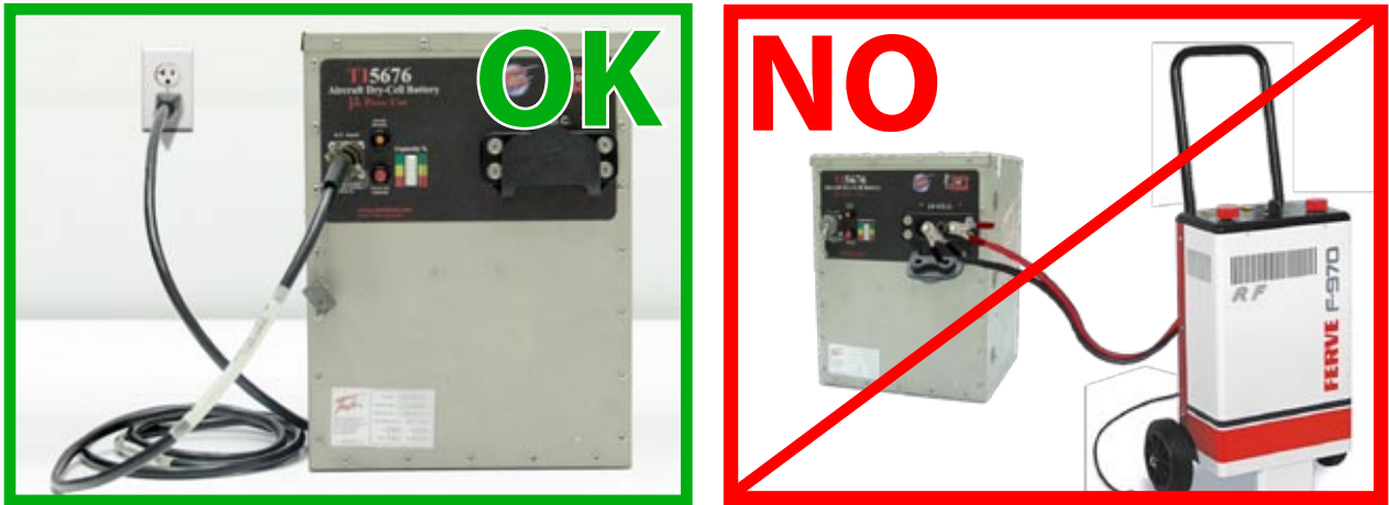
Figure 4.3.3 Proper and Improper Charging Methods
