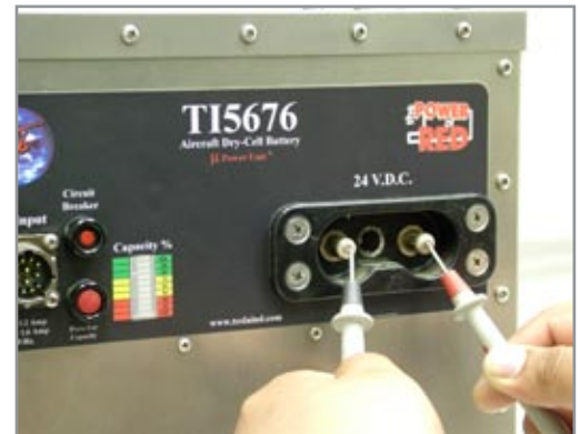
Figure 3.8.2 – Testing DC Receptacle
