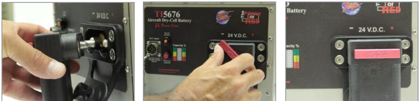
Figure 2.11.1 Attaching DC Power Cable to TI5676 MPU-24
