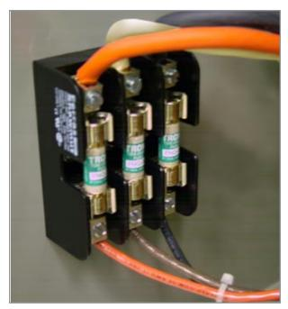
Figure 4.4.1 Replaceable Fuses
