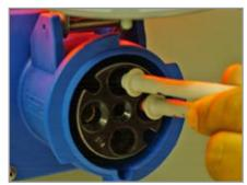
**1.** Move the negative probe to the upper phase 1 probe and the positive probe to right side phase 2 probe.
