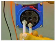
**3.** Move the positive probe to the lower phase 3 positive post.
