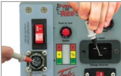
4. Move the positive probe to the dc negative post (A). Multimeter should read greater than 10 MΩ.
